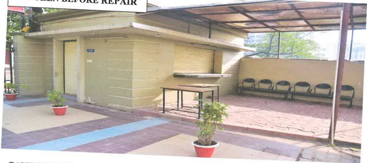
CANTEEN BEFORE REPAIR
